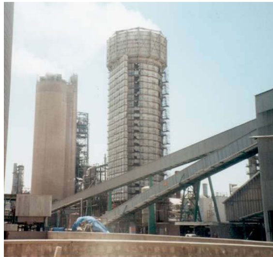
Figure 1. The Prill tower, shrouded with sheeting to control the bonding environment
