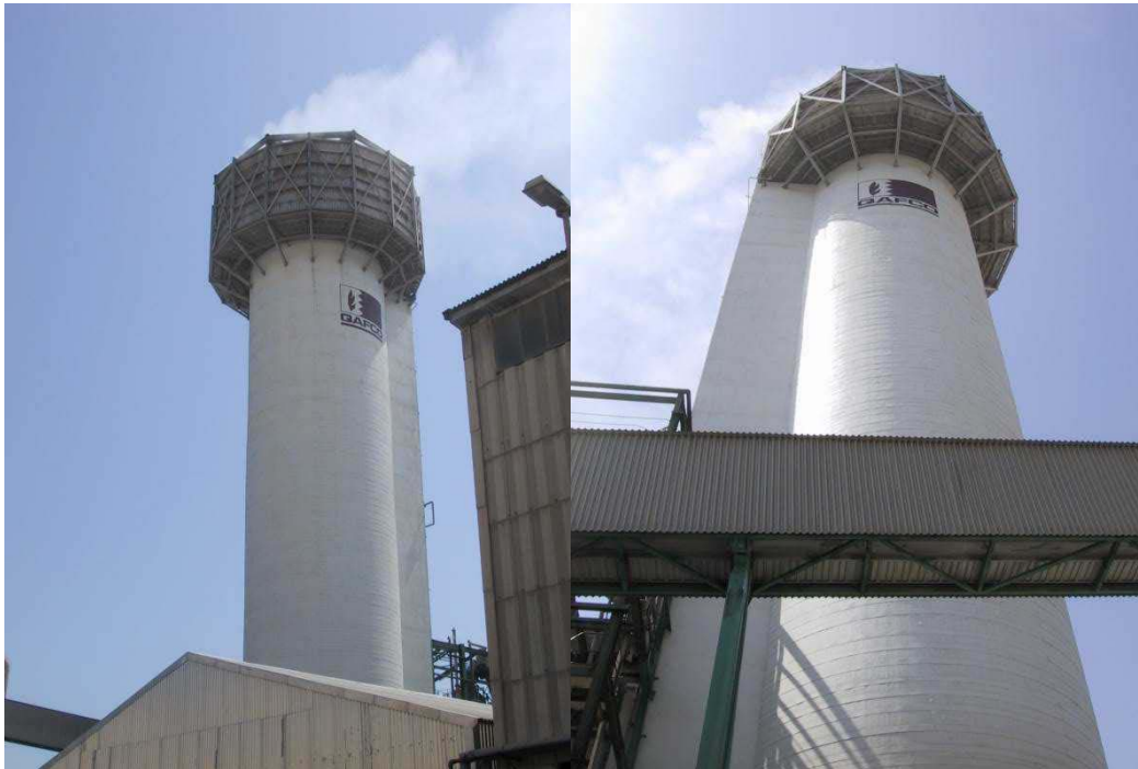
Figure 5. Strengthened and painted Prill tower
