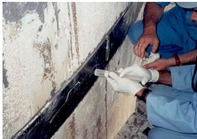
Figure 4. Checking and repairing voids
