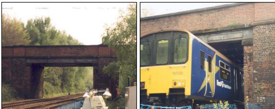
Figure 1. Approach photographs of New Moss Road Bridge
